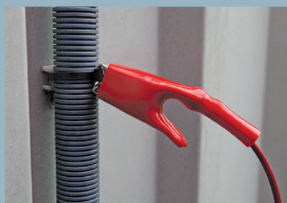
Small diameter cable tracing techniques
